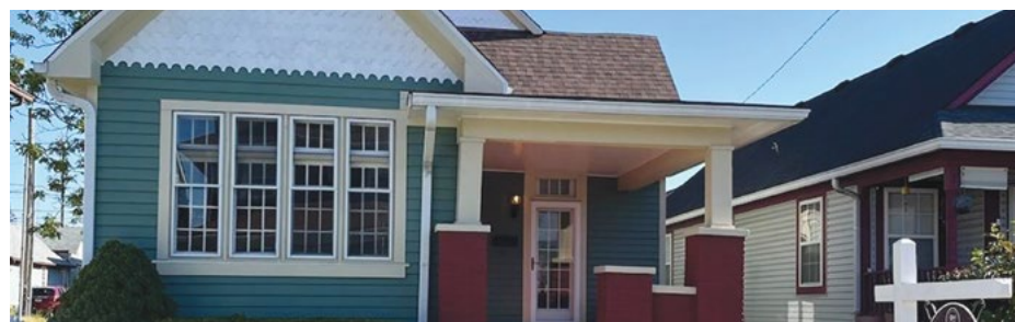
Historical home built in 1895 with fish scales and transom windows located in historical Ranson Place. Lots of parking in rear. Property sold as-is. NEW ROOF!
